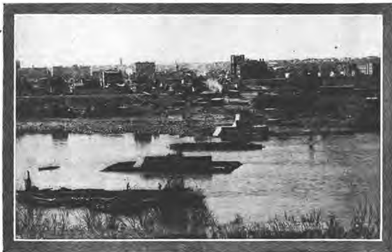
Ny bro under bygning i Saskatoon.
